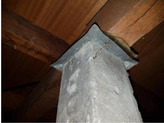
Brick veneer walls, constructed on brick strip footings, and with a suspended timber floor. There are concrete stumps in the subfloor, and the stumps are fitted with metal termite capping. Timber flooring, made from a hardwood. There is a concrete step, to the front of the building.
